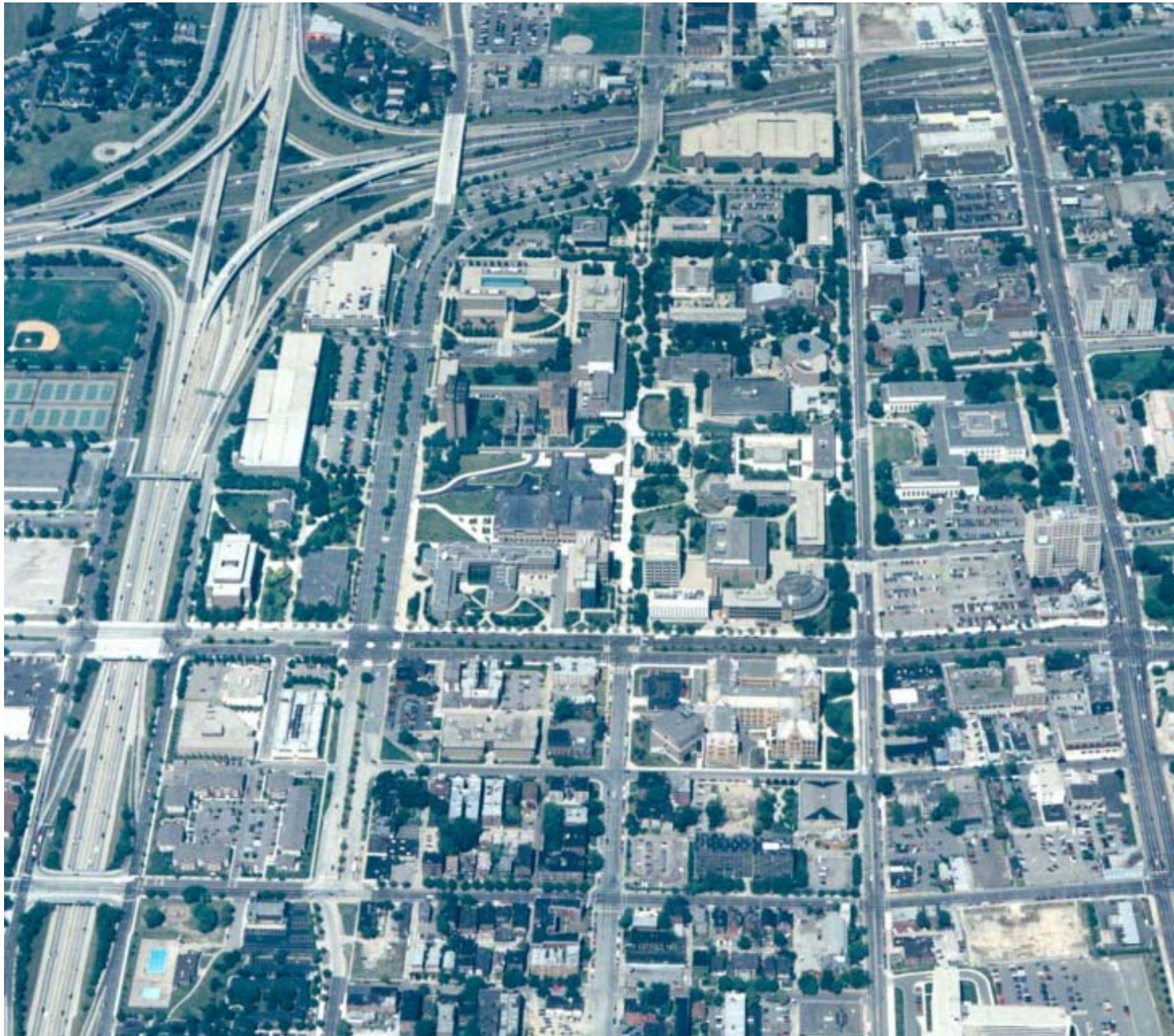
Aerial view of the central campus looking north
