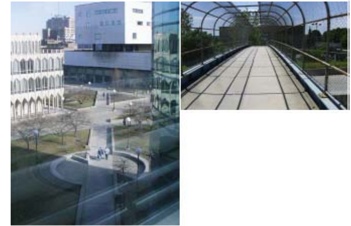
Connecting path to the Student Center Building, connecting pedestrian bridge to the Athletic Campus
