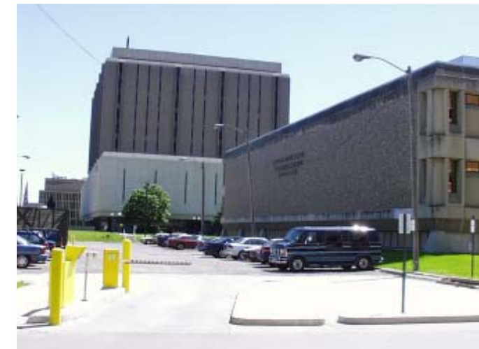
Shiffman Medical Library area dedicated to staff parking, building receiving and mechanical cooling towers
