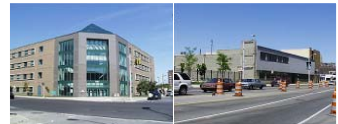
Academic Administrative Building, University Custodial Grounds Building
