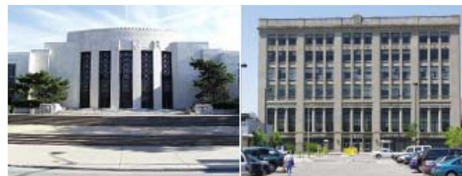
Horace H. Rackham Educational Building, Criminal Justice Building
