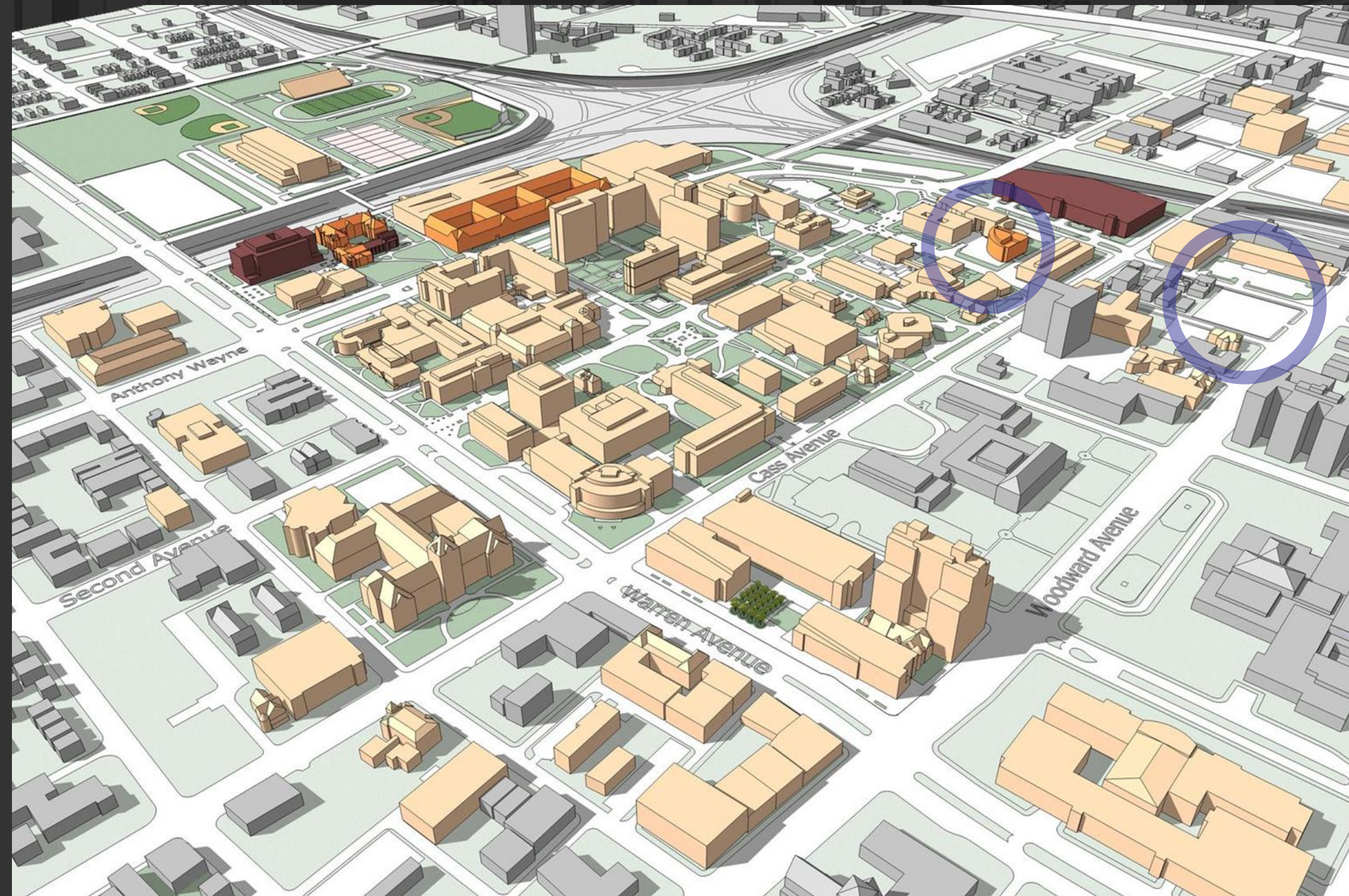
Main Campus View from Southeast
